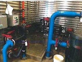
Water enters through the pipe on the West wall, goes upward and bends around pipe to the corner, then flows East through the County meter. 08/04/2015,E1571468.DOC2-EBRT 7119247
